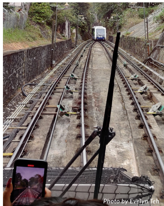
View from the front coach of the upgraded funicular train
