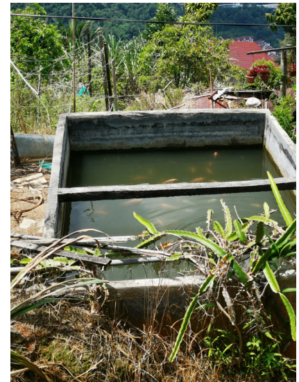
Pipes tapping water from further uphill and stored at retention ponds
