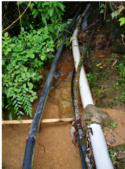
Pipes tapping water from further uphill and stored at retention ponds
